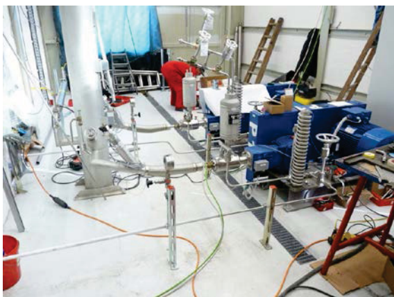
Figure 7: Refurbishment of GN2 station
