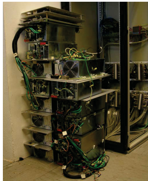
Figure 4: Replacement of obsolete MCC parts
